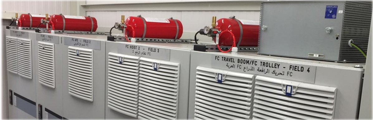
Fig. 1 R-DLP system protecting against fire in electrical control room switchgear of exported shipping container crane.
