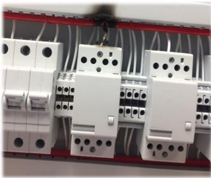
Fig. 2 - Ruptured tube at point of fire.
