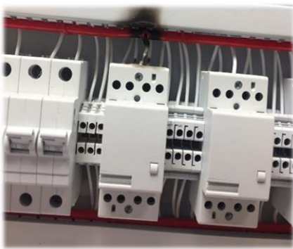
Fig. 2 - Ruptured tube at point of fire.
